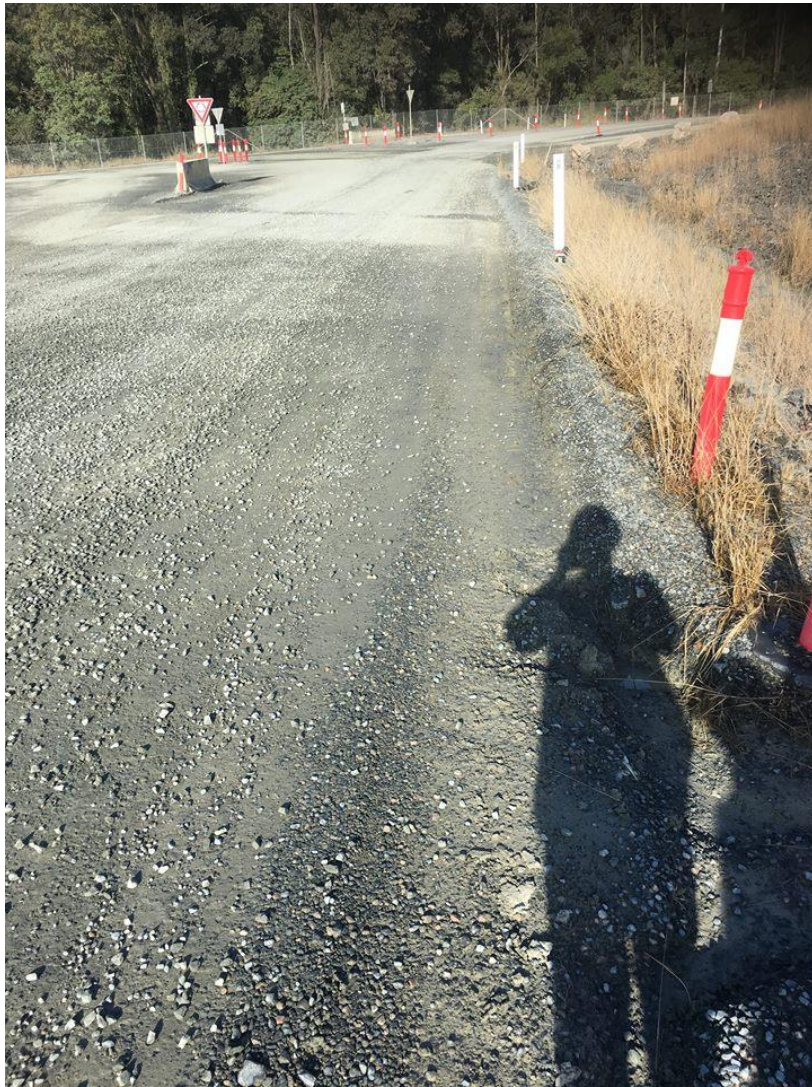
Figure 5. 4: Treated section of pavement facing South West on 23 August showing no major defects
