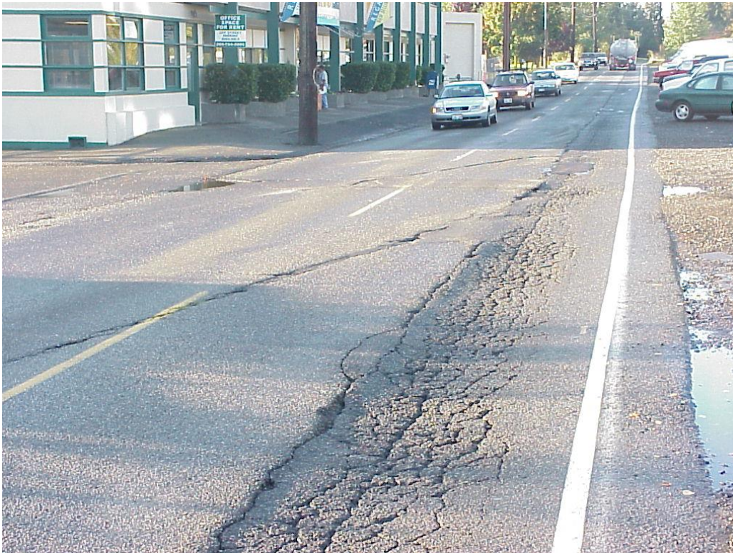
Figure 2. 2: Rutting and cracking of a pavement surface layer due to permanent deformation (Pavement Interactive 2018)
